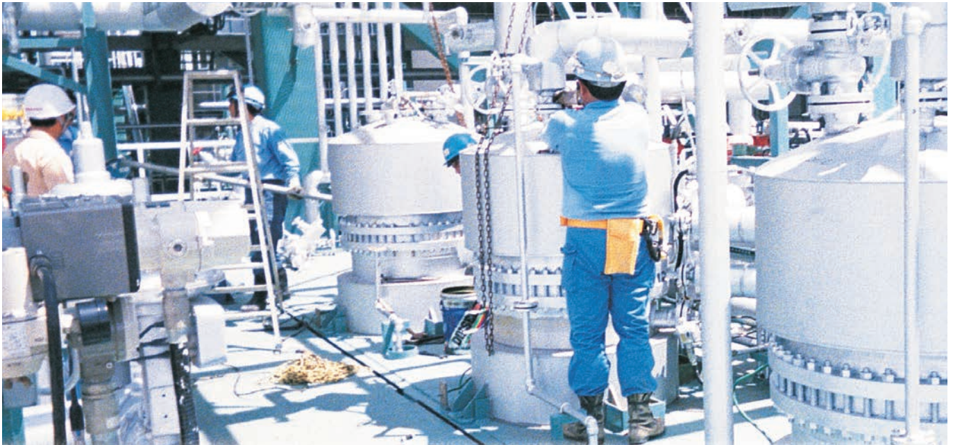
Refineries receive a high return on investment after installing Pall's backwash filters to protect catalyst beds and to remove catalyst fines from FCC slurry oil.
